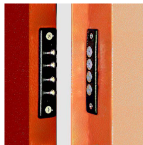
Electrical contacts between leaf and doorframe
