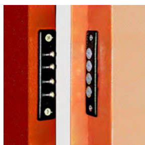
Electrical contacts between leaf and doorframe
